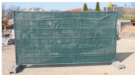
Figure 4: Example of a building site screen
