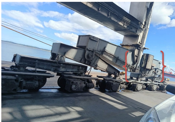
Picture 02: Leg 03- panel to be replaced
