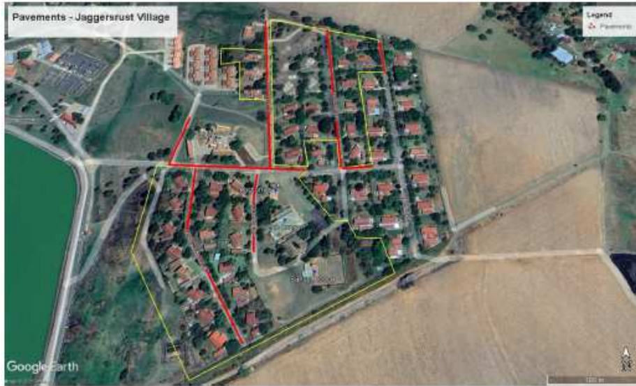
Figure 5. Pavement Maintenance at the Jagersrust Village
