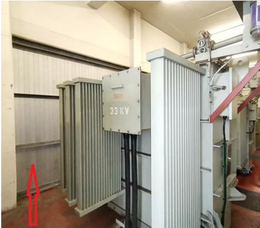
Figure 18: Transformer Room Roller door Openings
