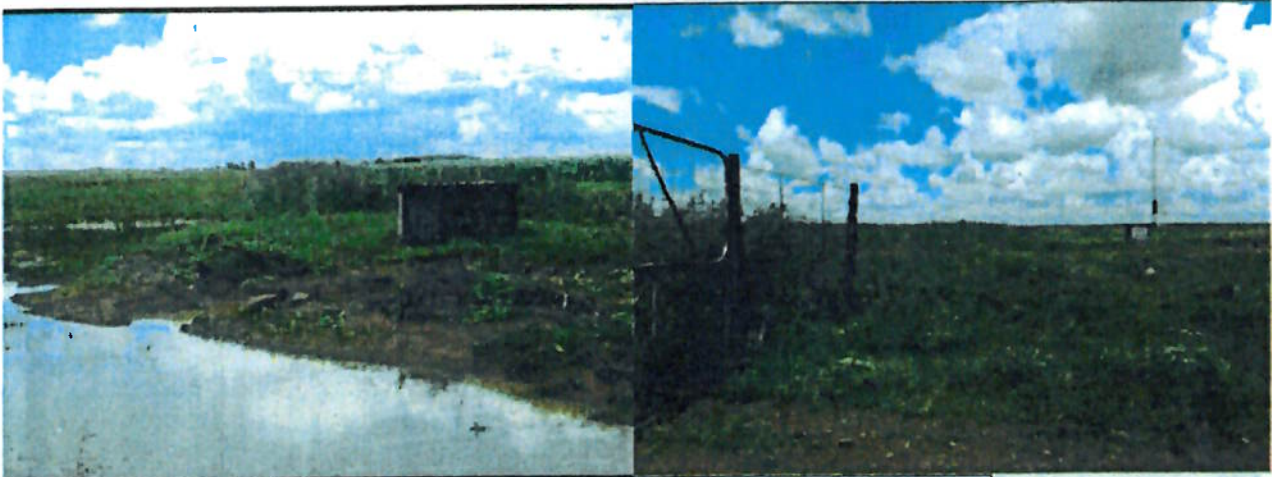
Pictures of the fence that was recently damaged by the flood
