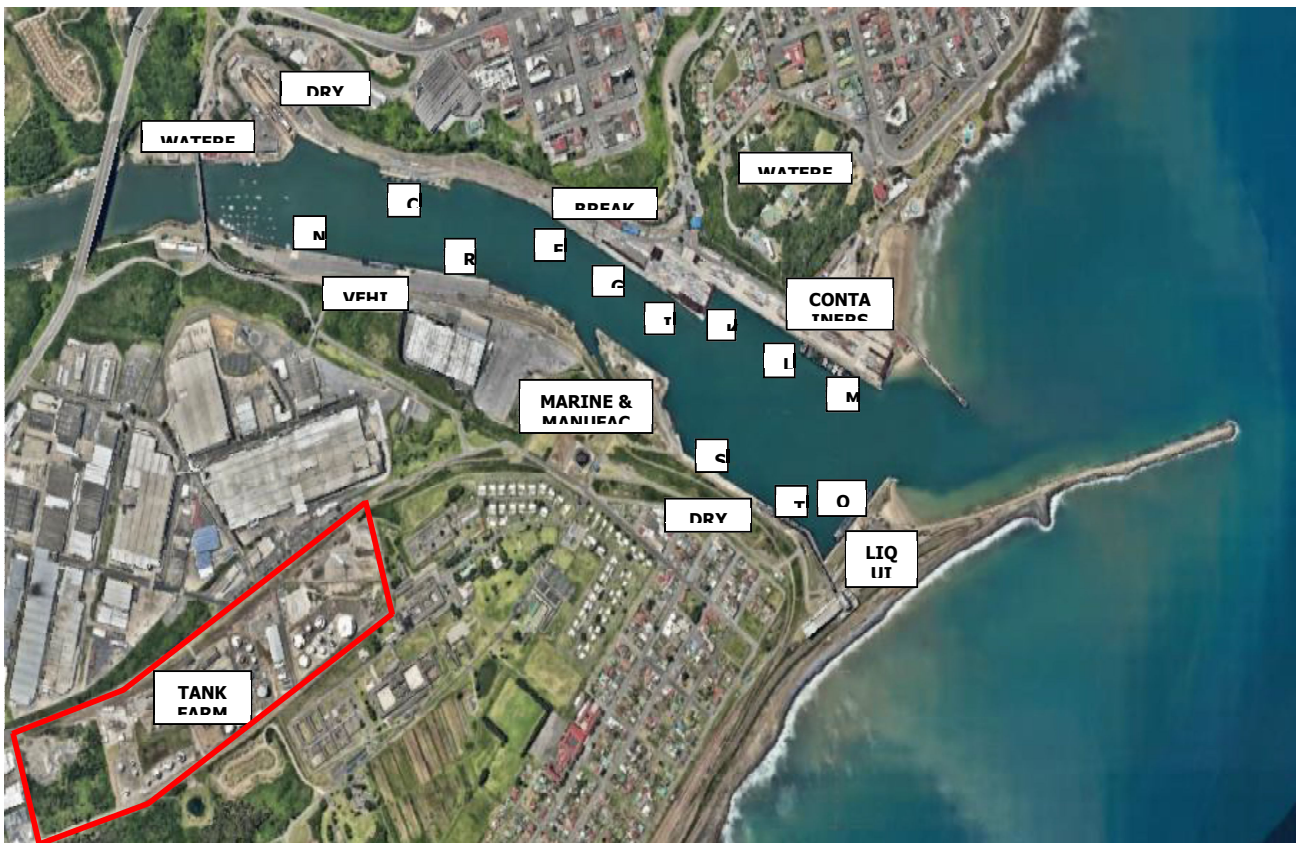
Figure 1: Port of East London
