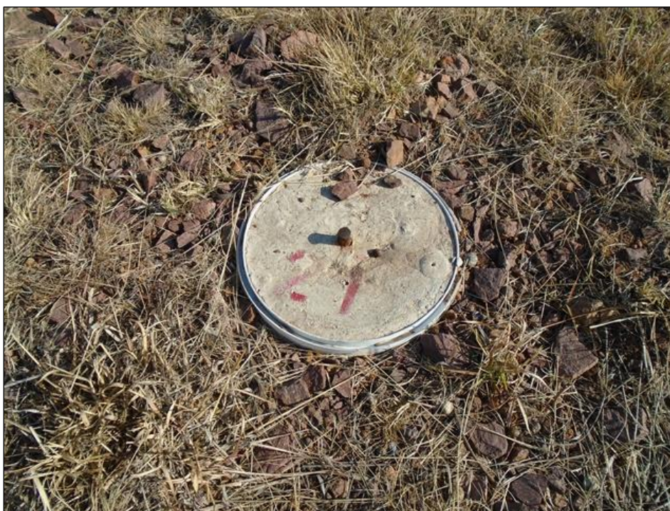
Figure 3: Settlement beacon typical example
