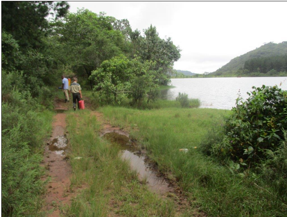
Figure 13: Condition of access road
