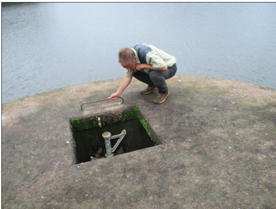
Figure 5: Access opening on top of intake tower
