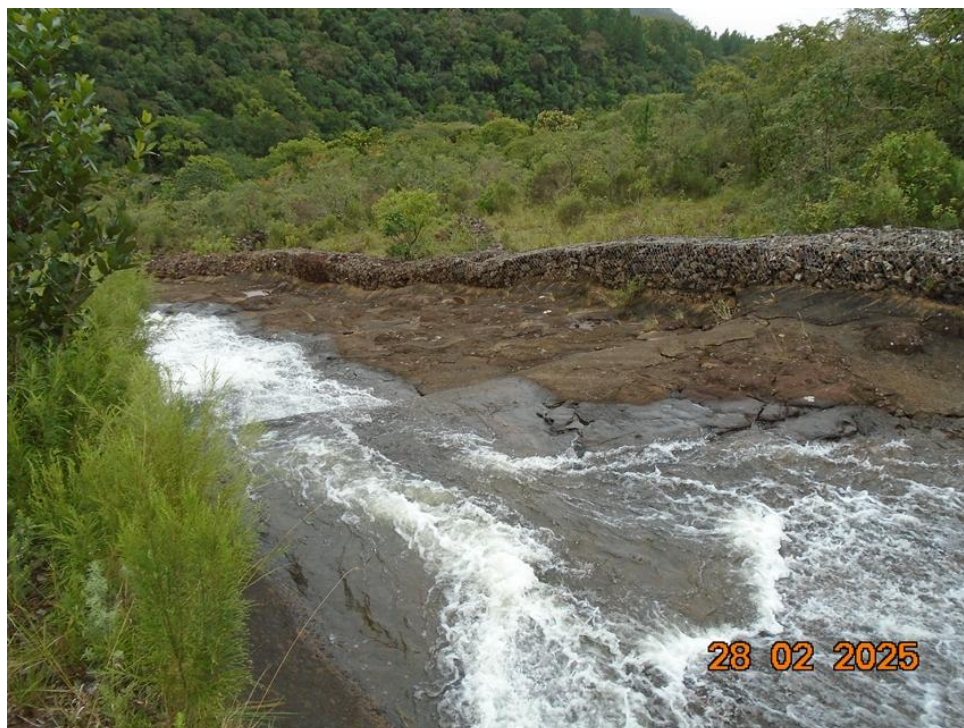
Figure 4: View of gabion side wall
