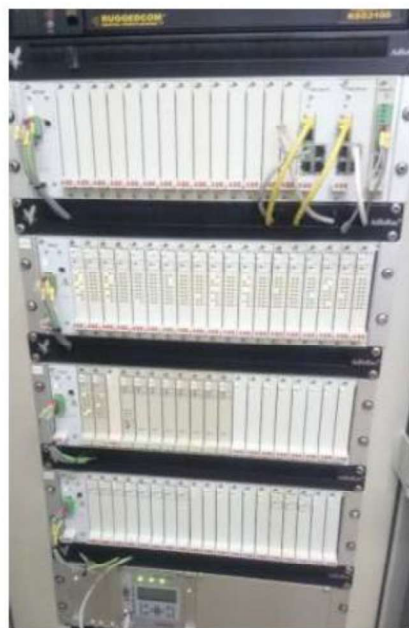
Photograph 38: System Control RTU Panel and Photograph 39: JLC & Electronic Governor of Unit 1
