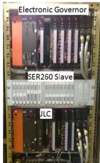
Photograph 38: System Control RTU Panel and Photograph 39: JLC & Electronic Governor of Unit 1
