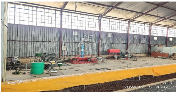
Figure 3: This picture shows the position of the area proposed for the WFTB relative to the sprinkler test bench
