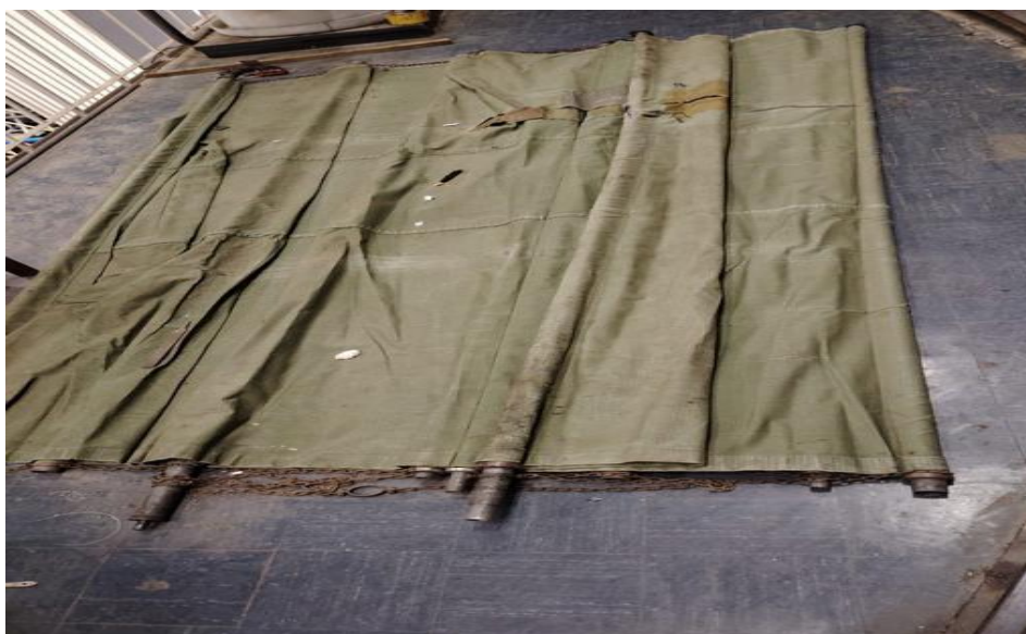
Figure 3: The existing windblind laid out on the floor (folded multiple times) showing the horizontal rails inserted into pockets along the length of the blind.
