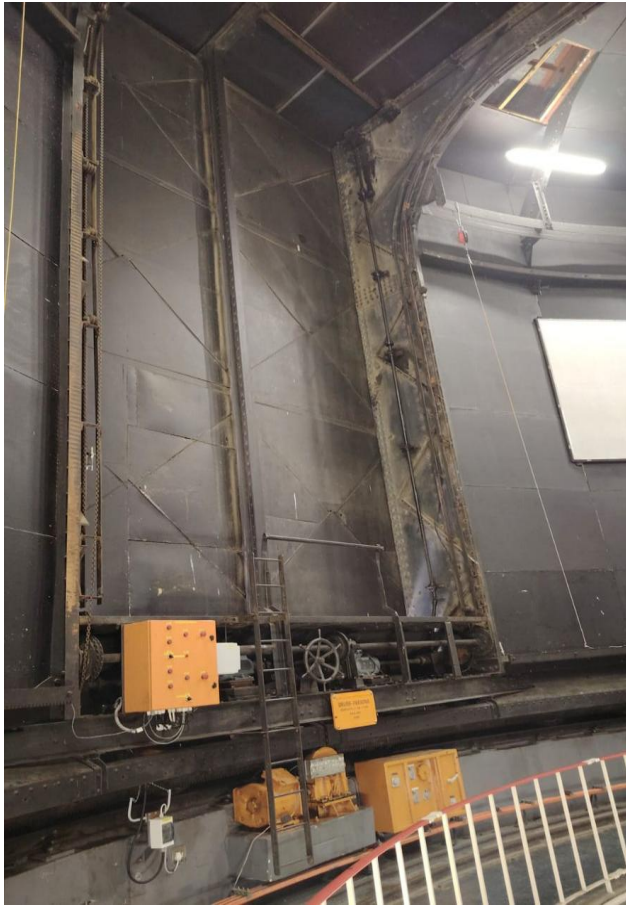
Figure 2: Left: The shutters in the 1.9-metre telescope's dome. When the windblind is fully raised, it covers the area indicated by the green rectangle. Right: When in the lowered position, the blind (green) folds and is stowed at the bottom of the shutters.
