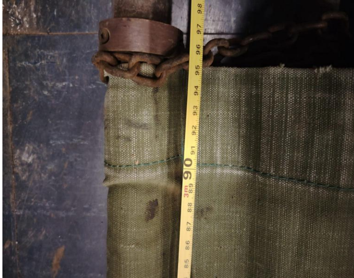
Figure 4: Close up of the existing windblind, showing the tough fabric required to withstand the force of the wind.
