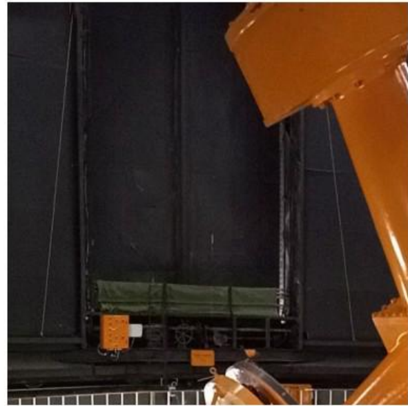
Figure 2: Left: The shutters in the 1.9-metre telescope's dome. When the windblind is fully raised, it covers the area indicated by the green rectangle. Right: When in the lowered position, the blind (green) folds and is stowed at the bottom of the shutters.
