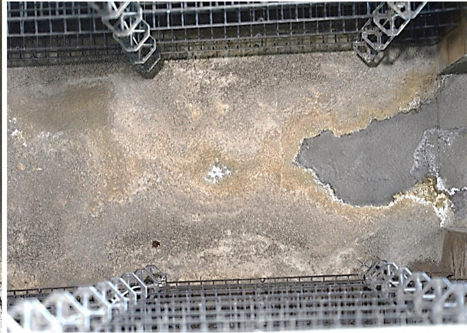
Figure 6: Sulphate Attack
