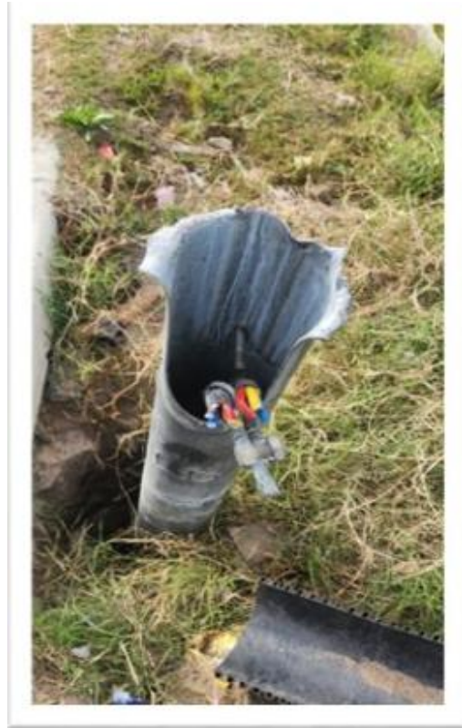
Picture 4 Streetlight Pole Cut
