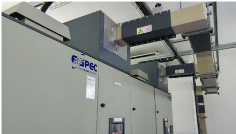
DPFC panel and overhead sealed bus bar controller
