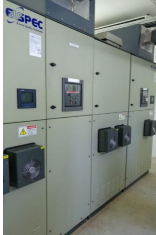
DPFC panel and overhead sealed bus bar controller
