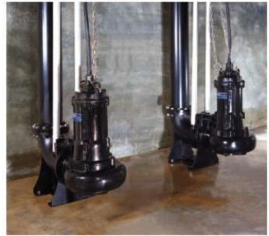
● Guide rail system installation
