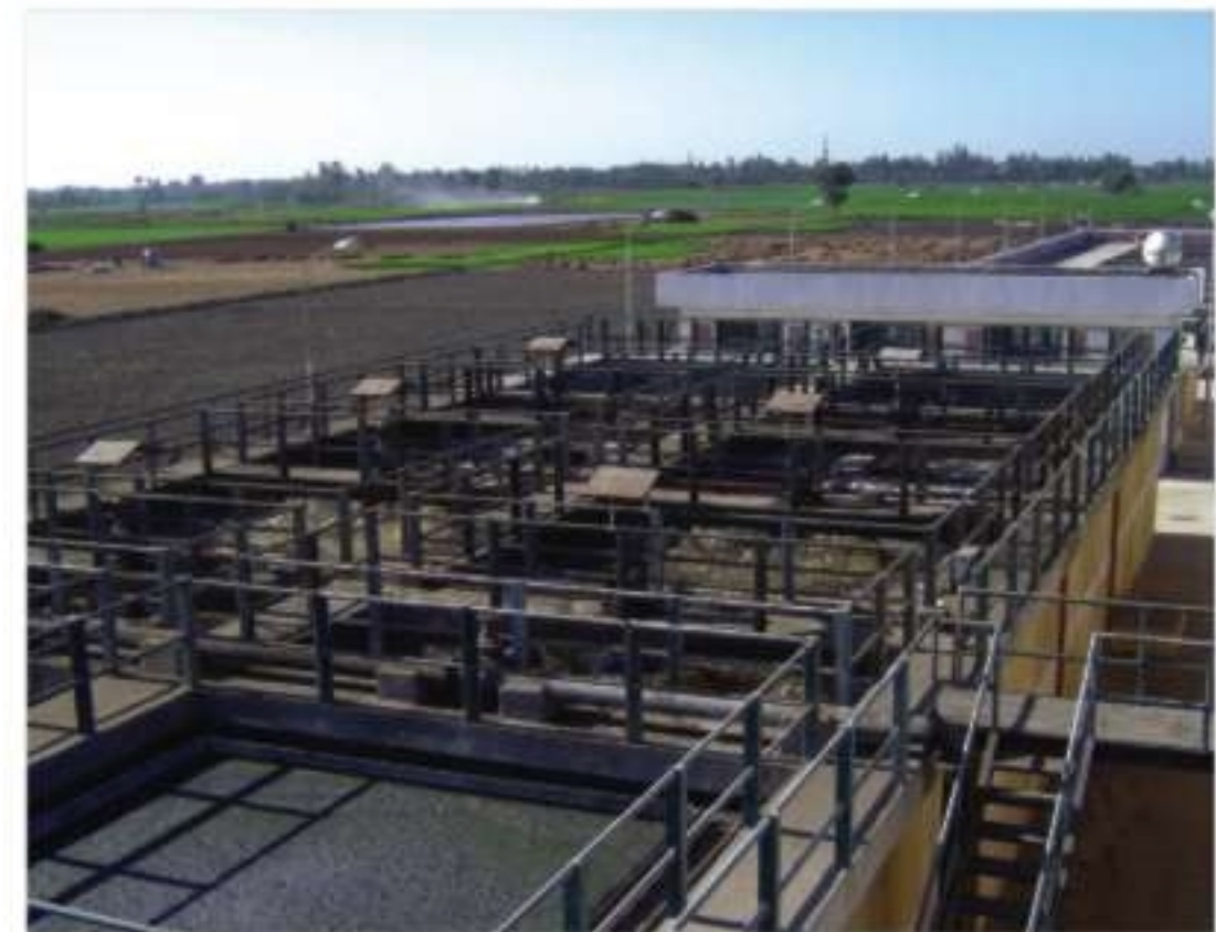
● Multi-drainage waste water treatment plant
