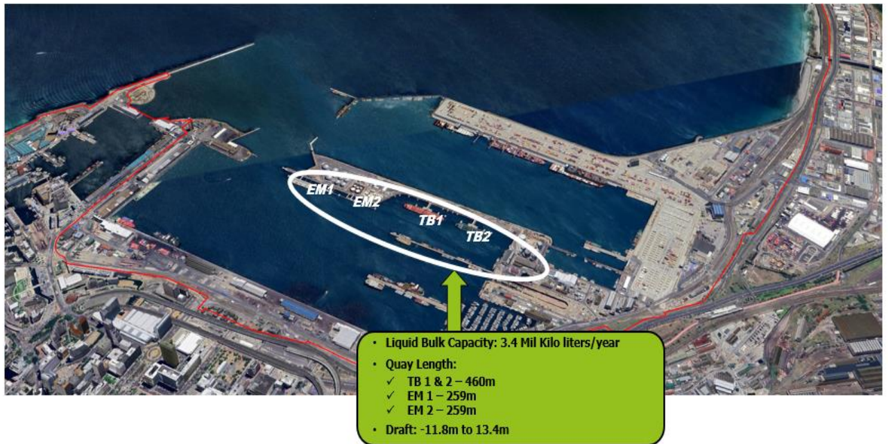
Figure 2. Aerial Overview of Liquid bulk Precinct
