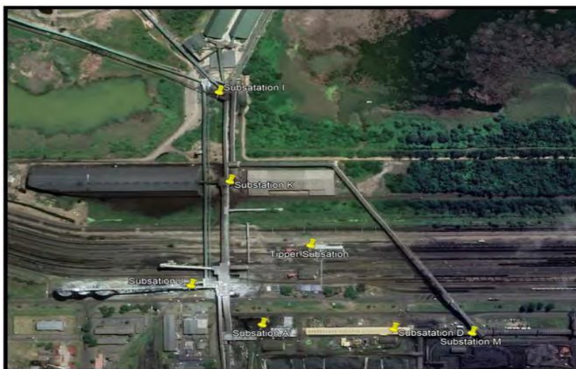
Figure 5 - Aerial Image 2: Substations Area View
