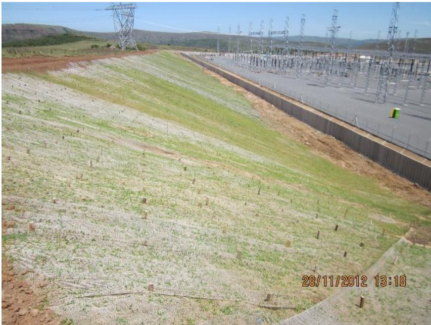
Embankment erosion control and a typical stormwater outlet
