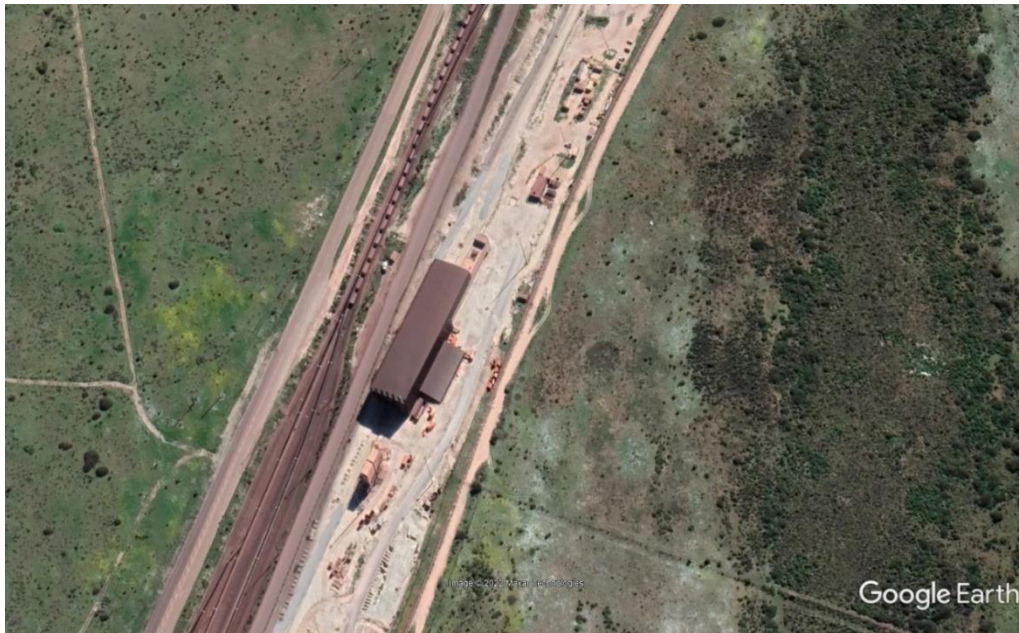
Figure 1: Aerial View of Tippler 3
