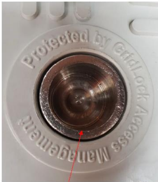
Spindle installed in manhole
