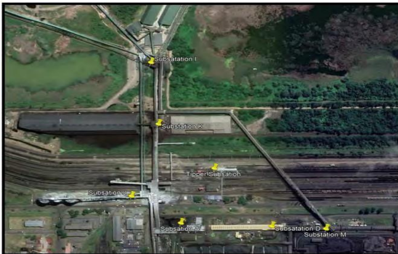
Figure 4 - Aerial Image 2: Substations Area View
