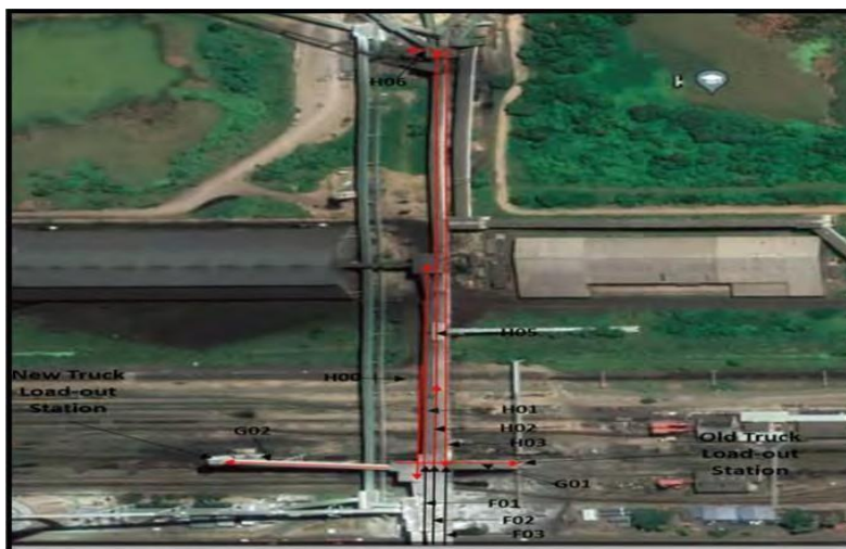
Figure 5 - Aerial Image 3: View of Conveyors and Galleries
