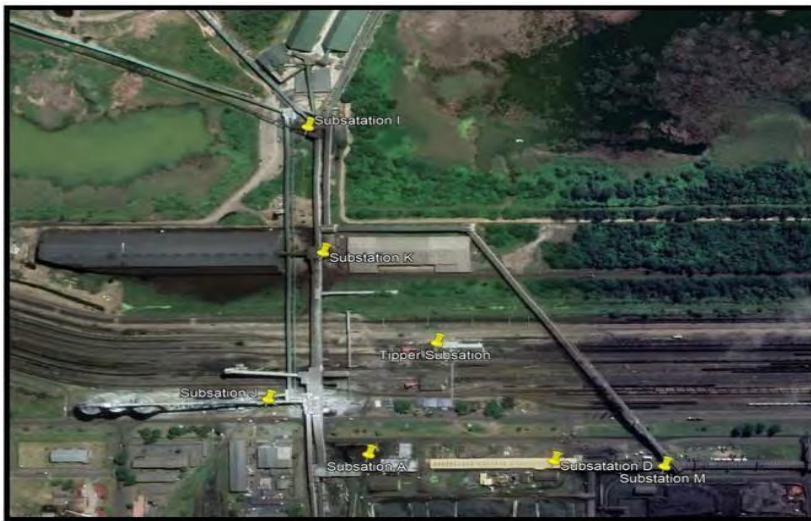
Figure 4 - Aerial Image 2: Substations Area View
