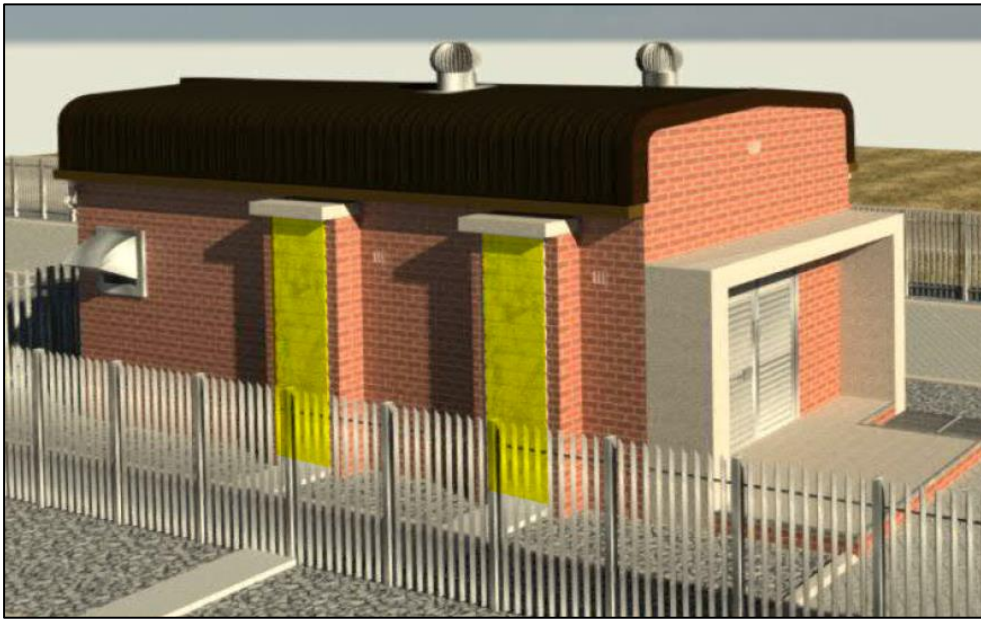
Figure 79: Cable ducts highlighted on exterior
