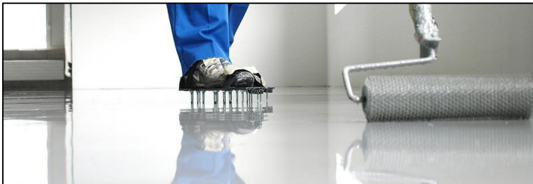
Figure 73: Typical Sikafloor installation
