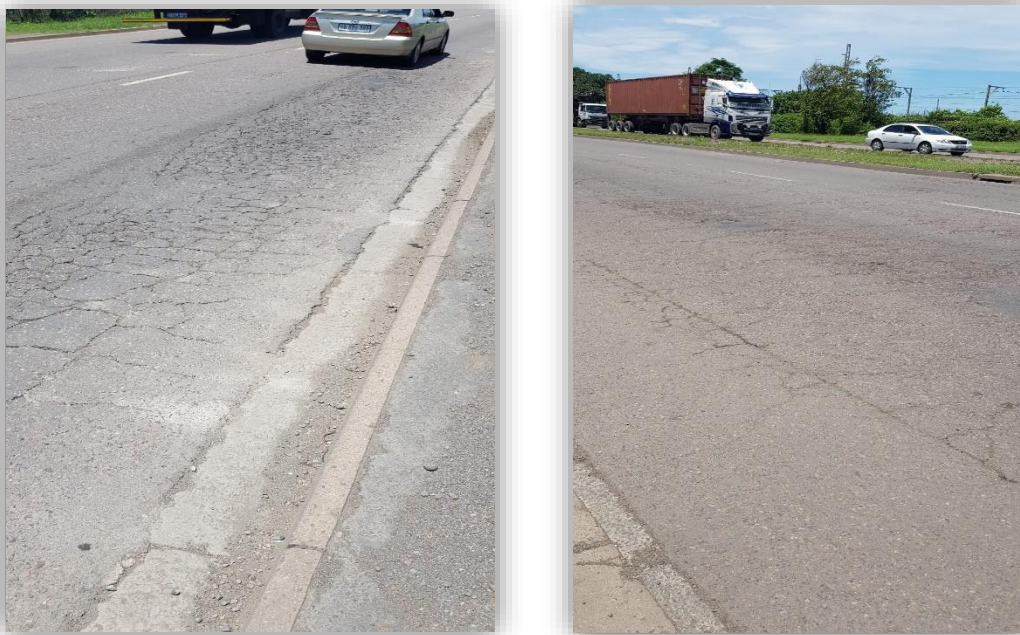
Figure 8-1: Crocodile & Rutting on Bayhead Road
