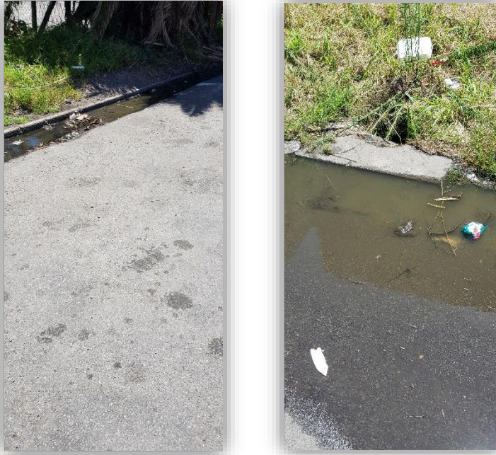
Figure 8-4: Water ponding, blocked and overgrown drainage channel at Langeberg Road
