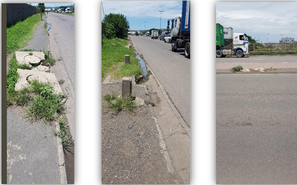
Figure 8-2: Damaged Kerb Inlets at Bayhead Road
