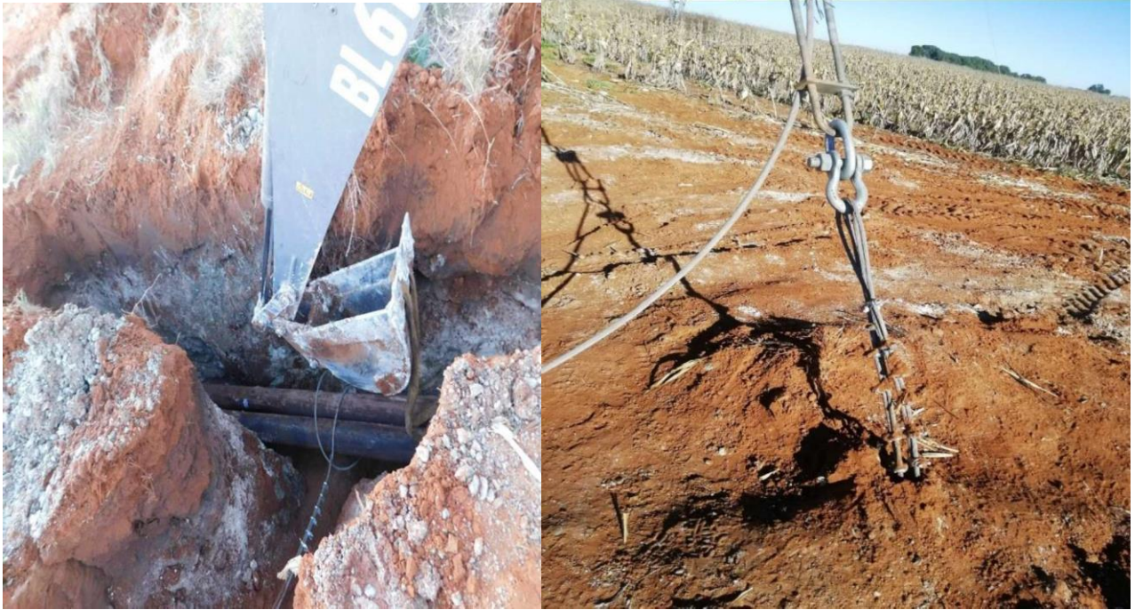
Figure 2: Temporary Wooden Poles
