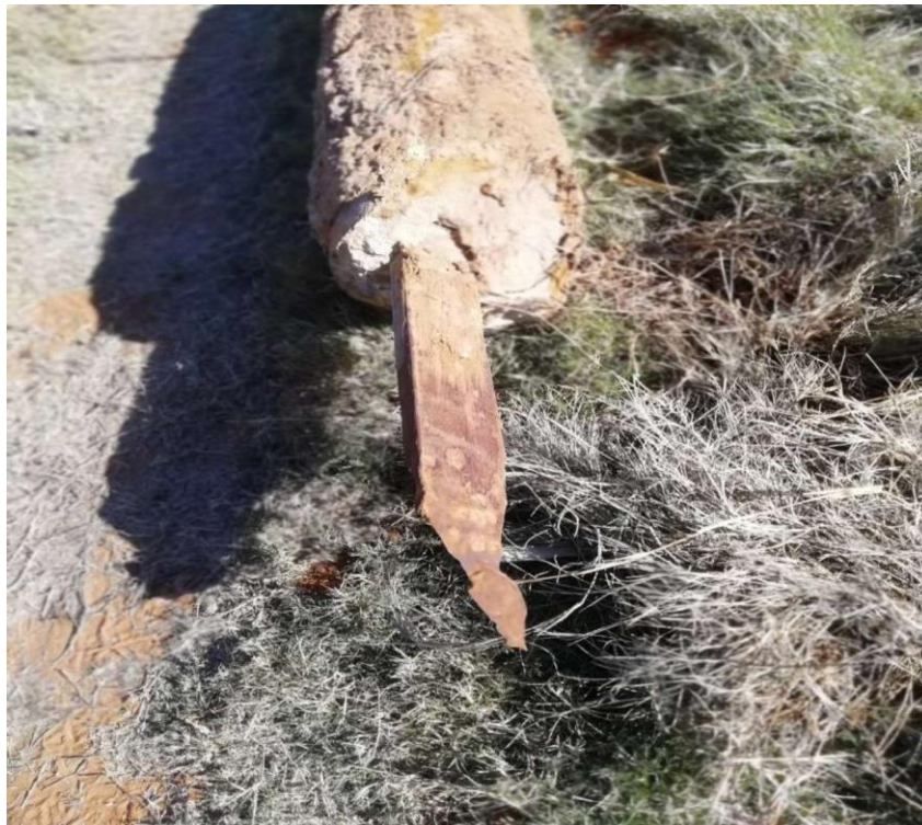
Figure 3: Section of the guy anchor that pulled out
