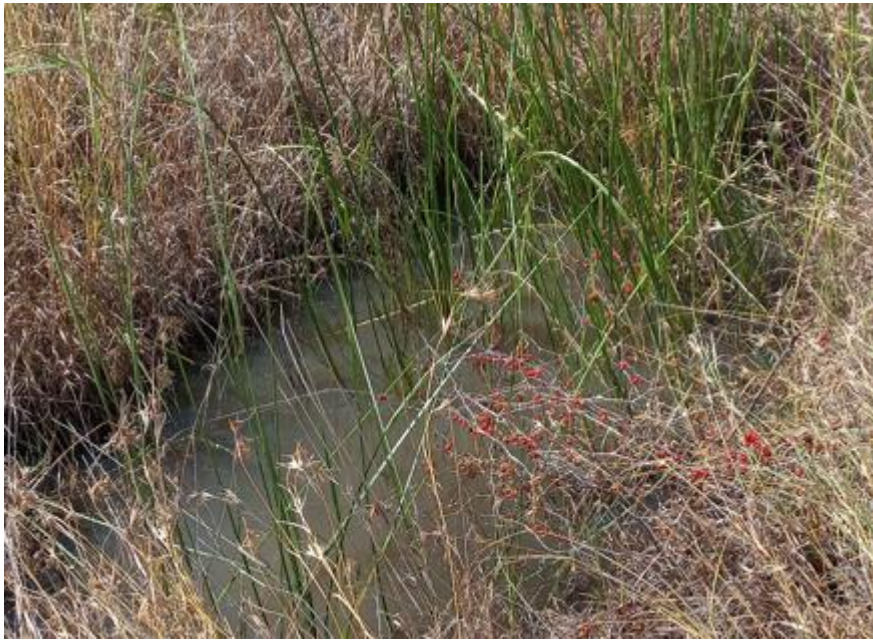
Figure 9: Ponding of water by existing guy anchor links
