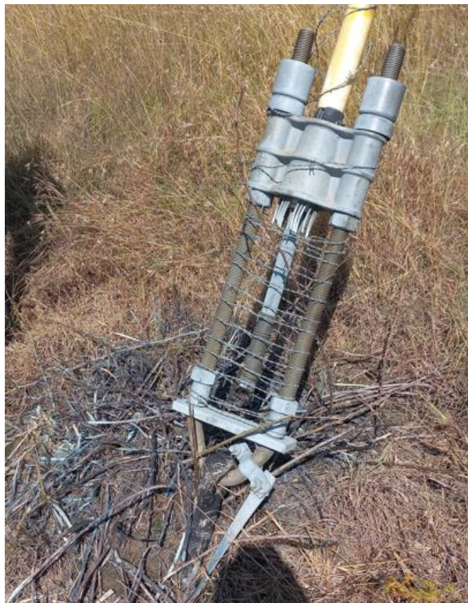
Figure 8:Existing guy anchor
