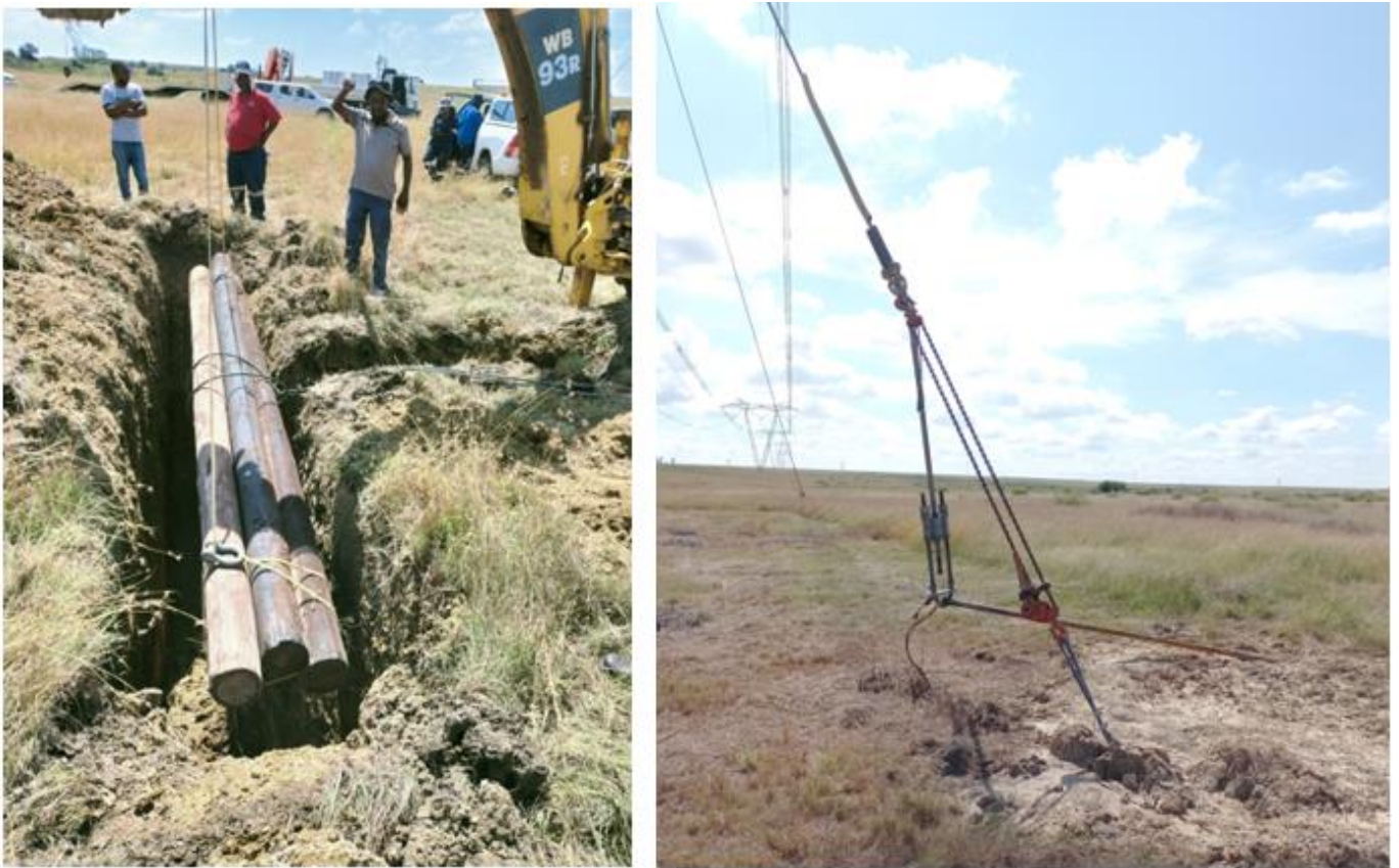
Figure 11: Temporary backstay
