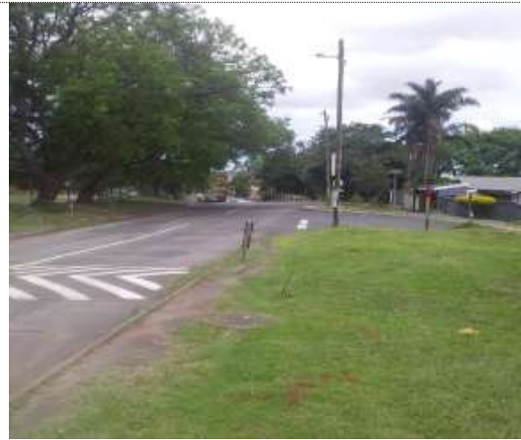
Photo 8 – Existing overlying electrical cables along the proposed site area.
