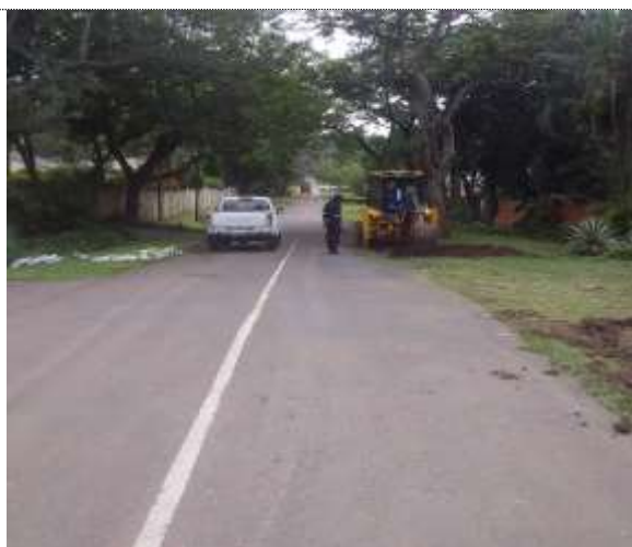
Photo 2 – Test Pit Excavation on Amersham Road.
