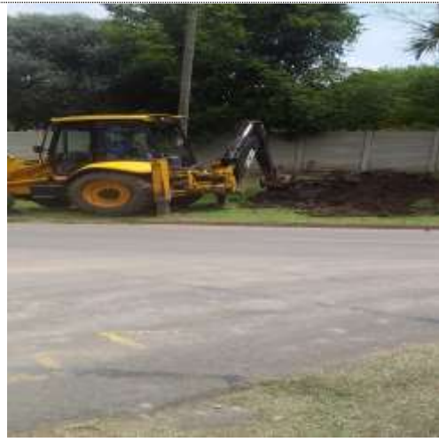
Photo 5: Trial Pit excavation on site.
