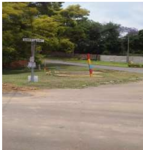
Photo 2 – Existing Pipeline Markers on Amersham and High Wycombe Road.
