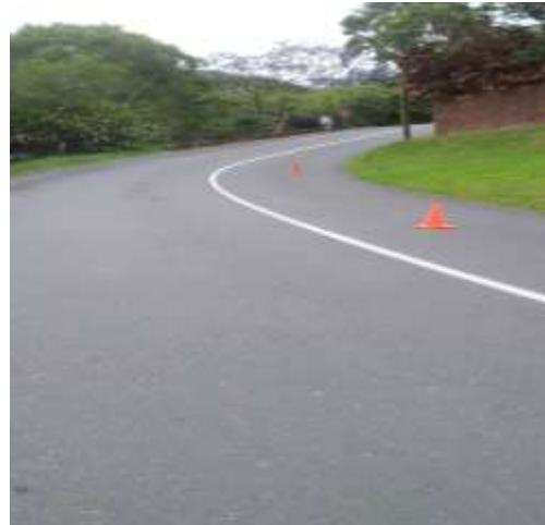
Photo 8 – Marlowe Road closely adjacent to the proposed pipeline WP#4.
