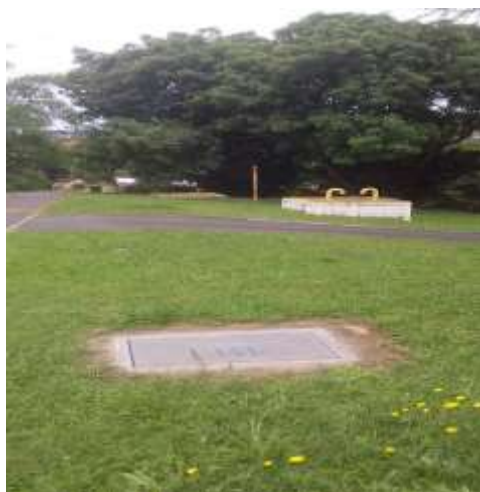
Photo 1 – Existing Water Chambers on Amersham and High Wycombe Road.
