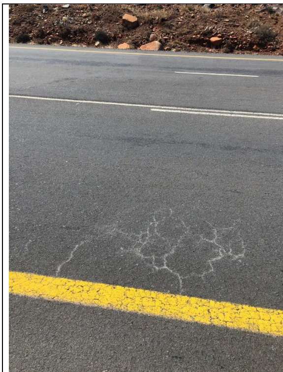
Rutting, Crocodile cracking, pumping
