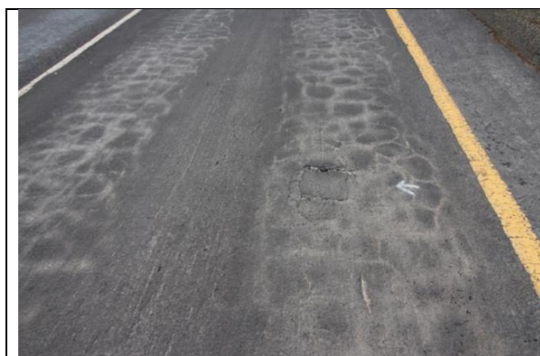
Rutting, Crocodile cracking, pumping
