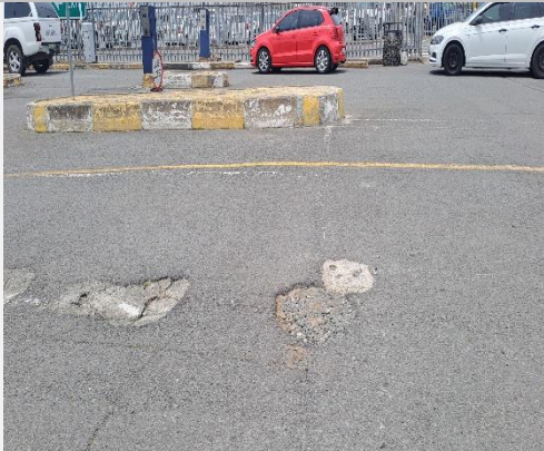
Figure 11: Opposite Guard House (7mx1.5m)
