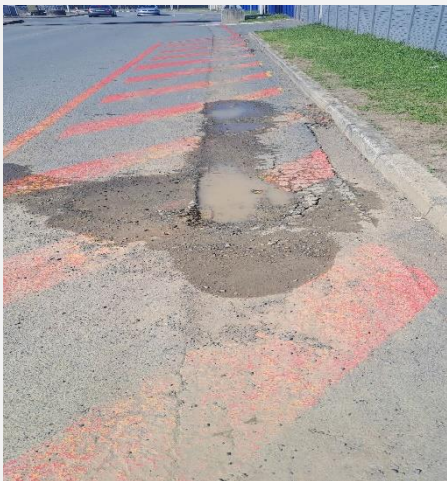
Figure 12: Next to Europcar (7mx0.2m), Investigate, repair on a 32mm water pipe.
