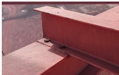
Counterweight frame structural connection
