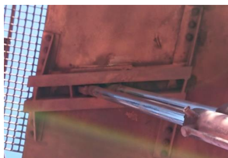
Operators cab luffing cylinder upper connection bolts
