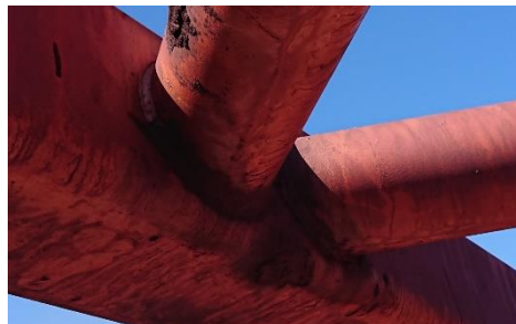
Boom upper support structure connection
