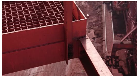
Mast walkway stanchion connection
