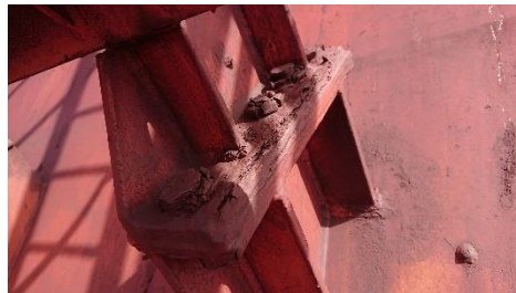
Mast walkway connection
