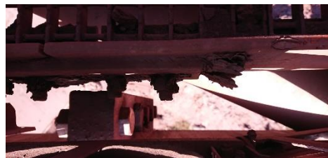
Boom walkway structure splice connection
