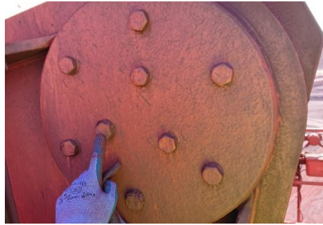
Luffing cylinder lower pivot connection
