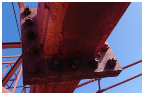
Boom upper support structure connection
