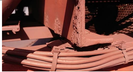
Mast walkway connection
