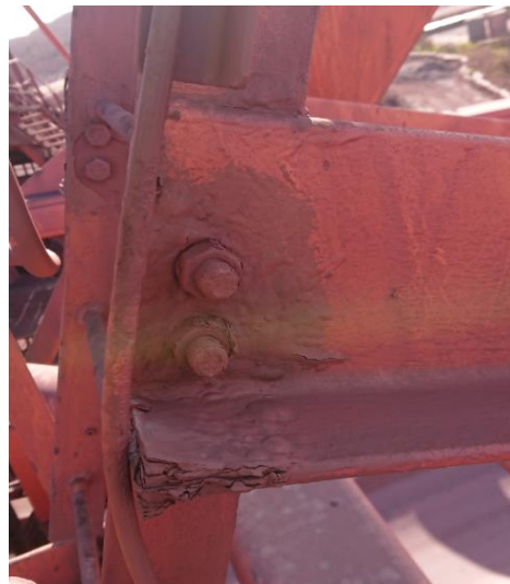
Jackstay lower catladder connection
