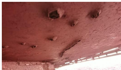
Underside of slew deck
