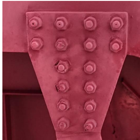
Underside of gantry
