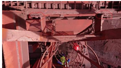
Mast catladder connection
