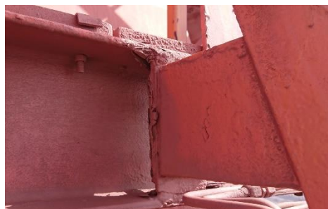
Mast walkway connection
