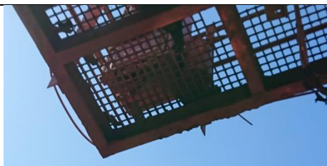
Operators cabin support structure
