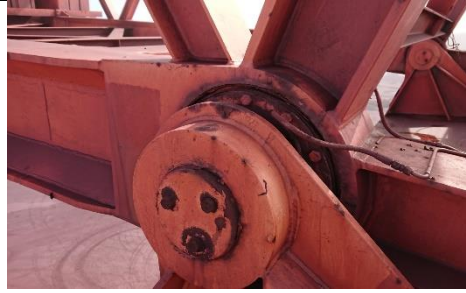
Counterweight frame pivot connection
