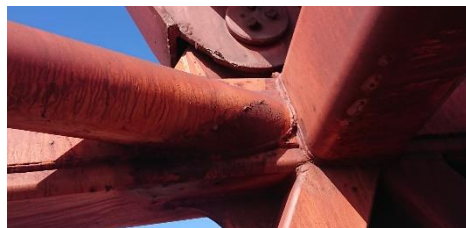
Boom upper support structure connection
