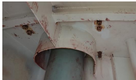
Slew drive mounting bolts
