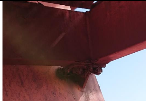
Mast walkway connection
