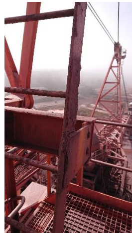
Counterweight frame catladder connection
