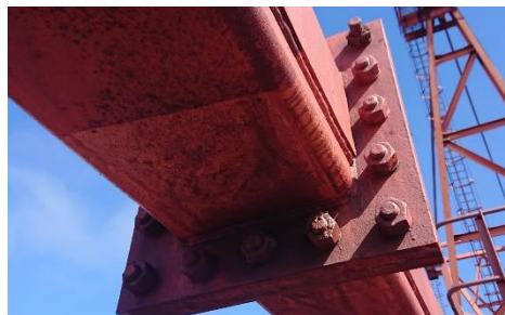
Boom upper support structure connection
