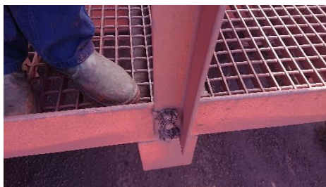
Boom walkway stanchion connection
