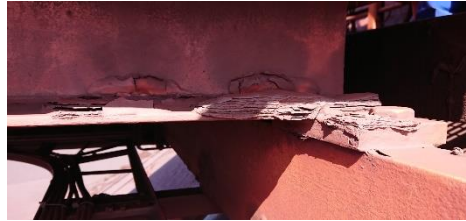
Mast walkway connection
