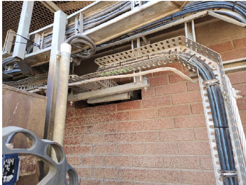
Figure 2: Typical Cable Tray entry
