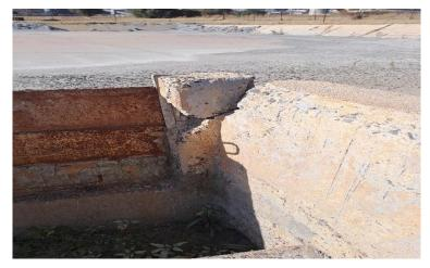
Repair of the 0.5 m X 0.3 m X 0.3 m along with the rebars
