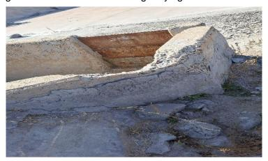
➤ Surface concrete repairs (0.2 m X 0.3 m X 0.3 m) along with rebars
