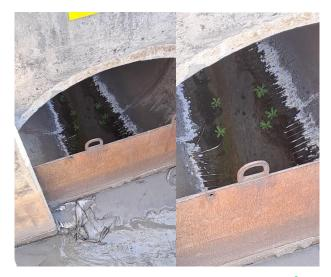
➤ Surface concrete repairs, estimated total area = 15m² including rebars
