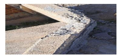
Surface concrete repairs (0.2 m X 0.3 m X 0.3 m) along with rebars
