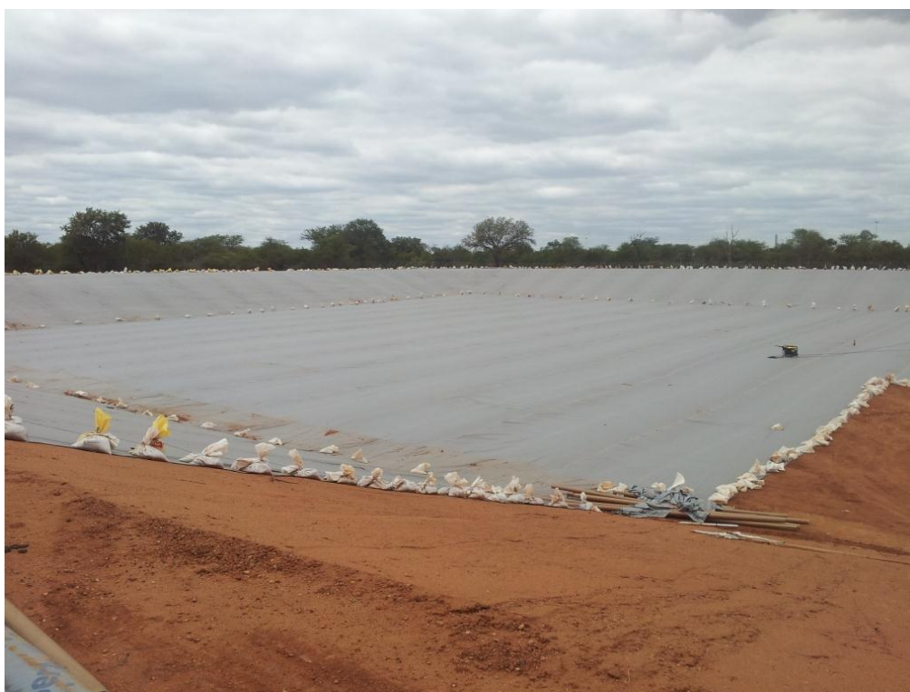
Figure 2.2: Example of a typical lined pollution control dam
