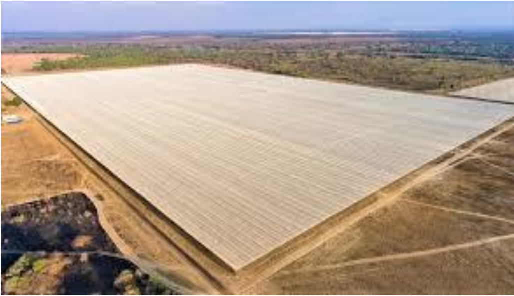
Figure 3: Aerial view of a similar Structure
