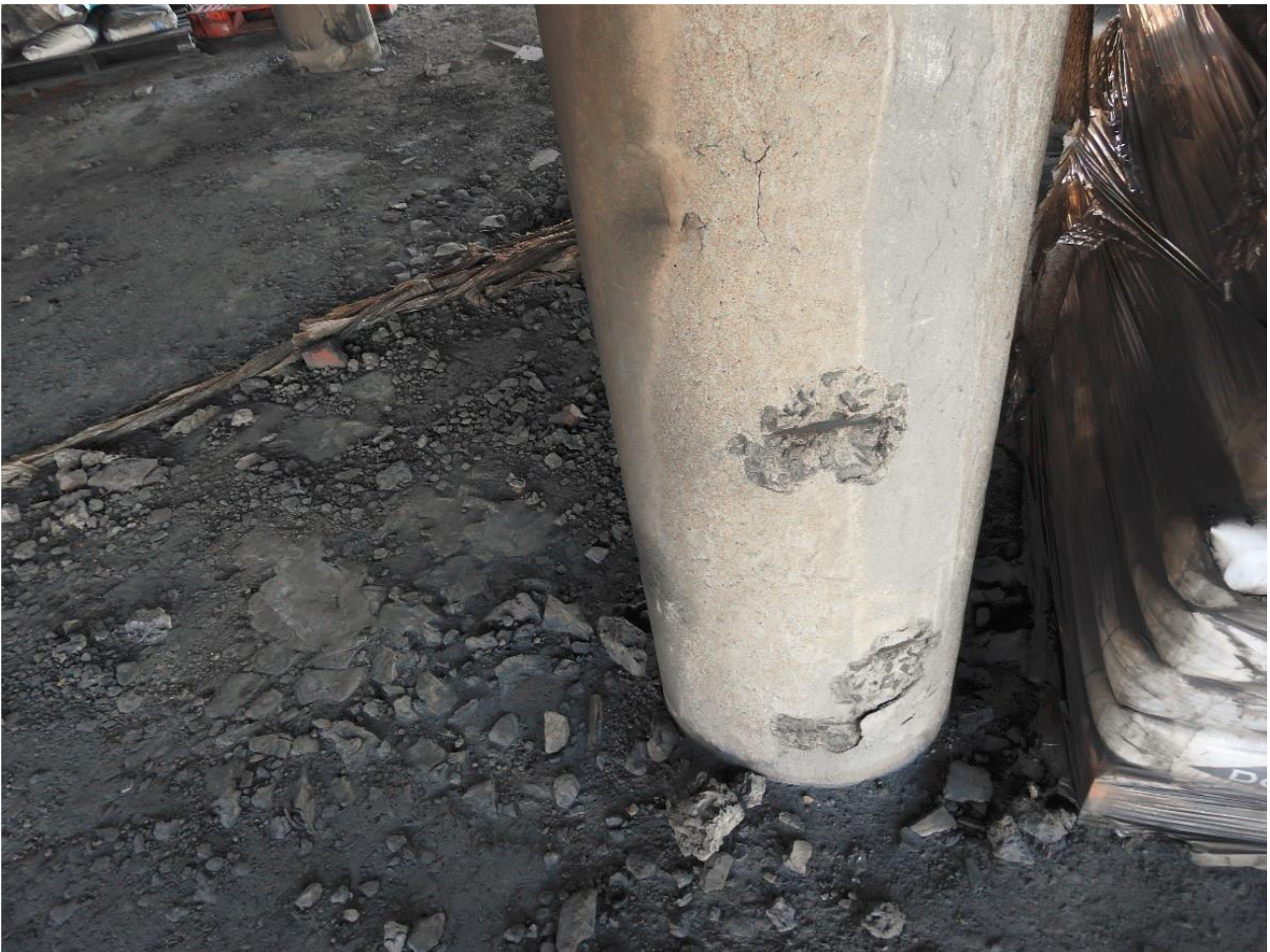
Figure 3: Circular columns for clarifiers
