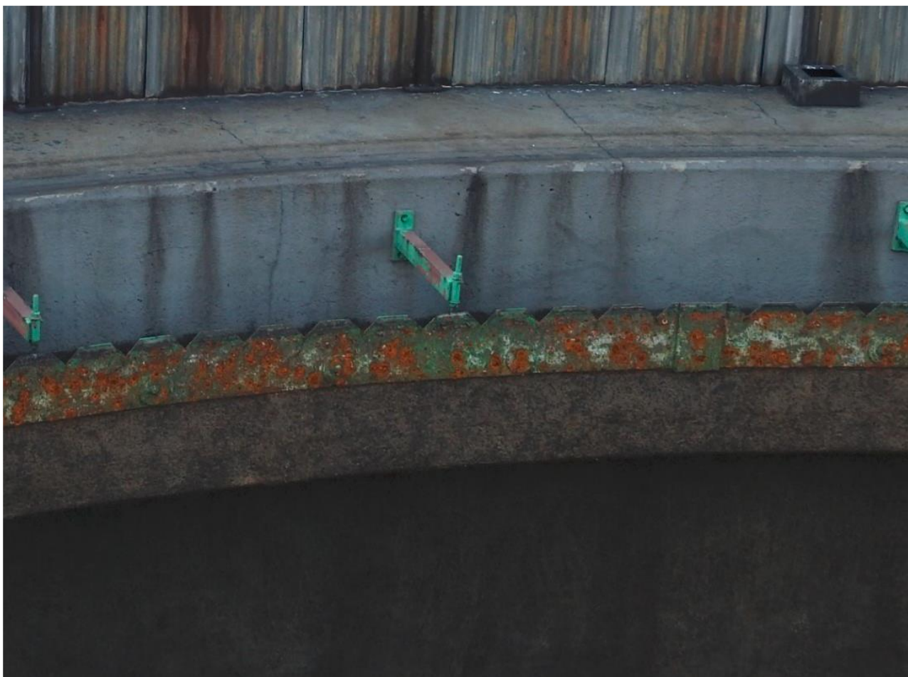
Figure 2: Internal structure for clarifiers
