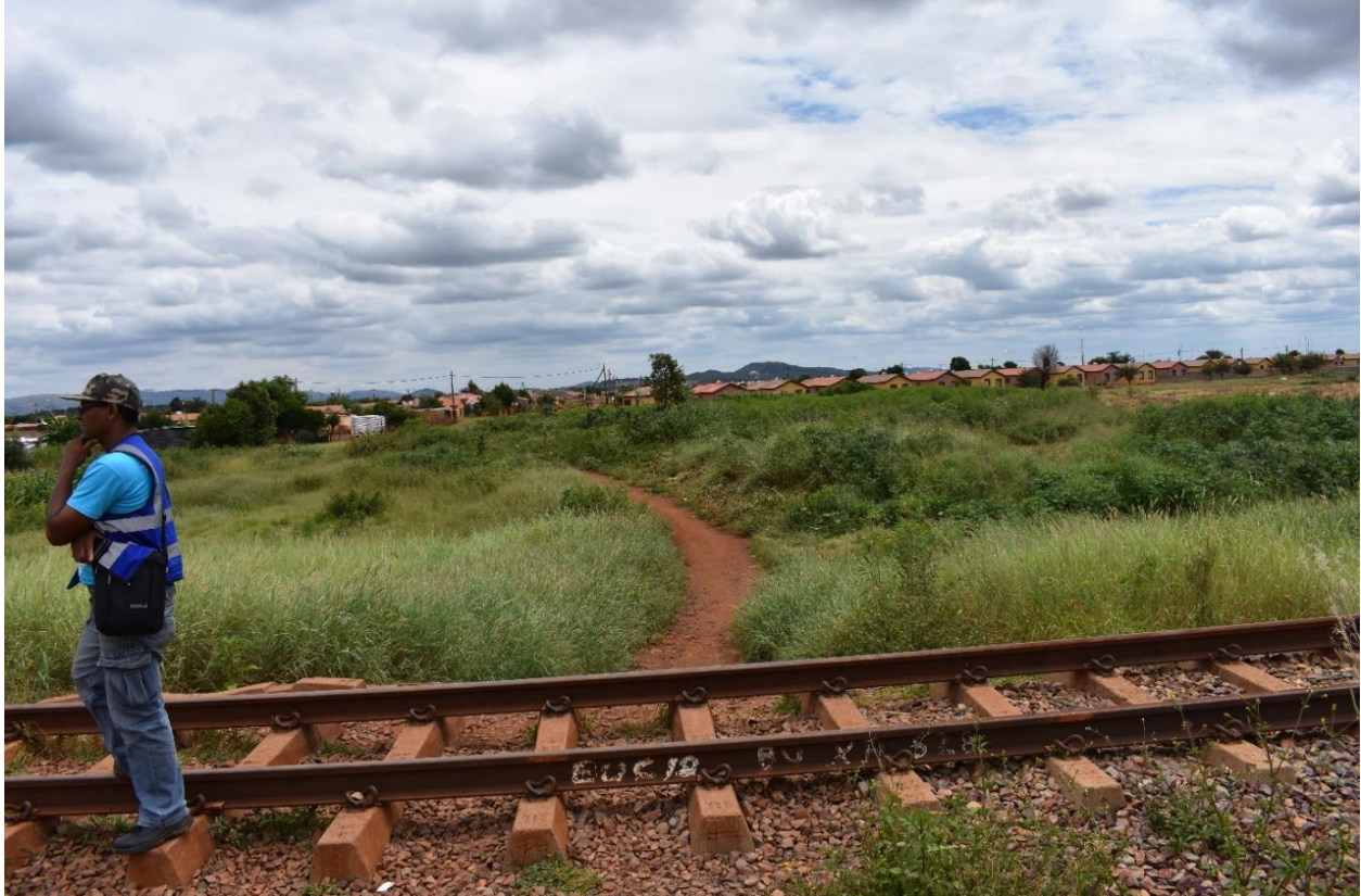
Figure 4: Bridge 6 - Footpath leading away from the rails.
