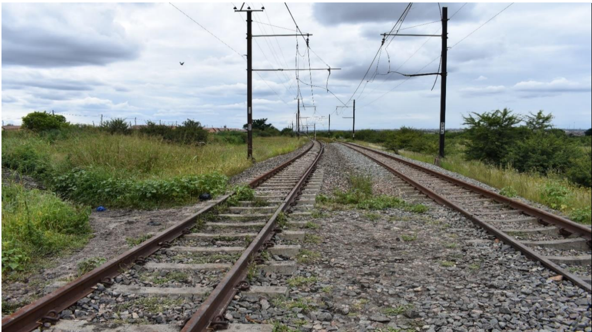
Figure 9: Bridge 8 - Track leading to illegal tracks crossing.
