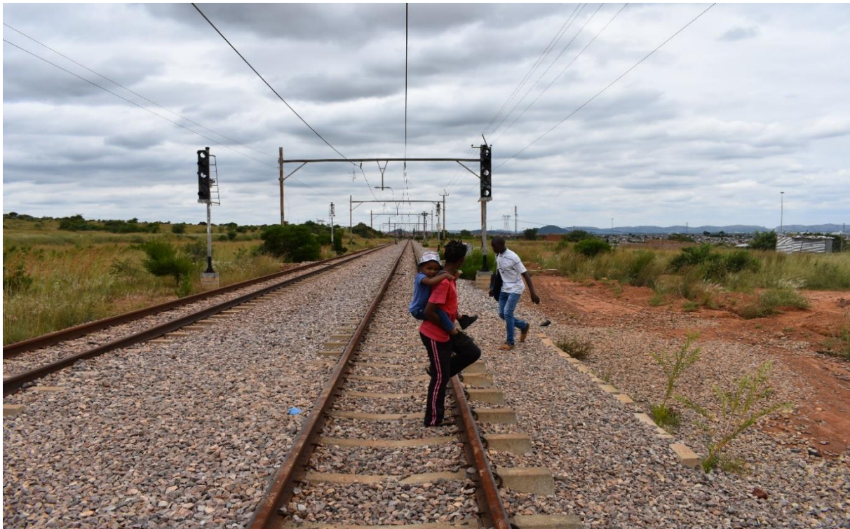
Figure 3: Bridge 5 - Crossing tracks illegally
