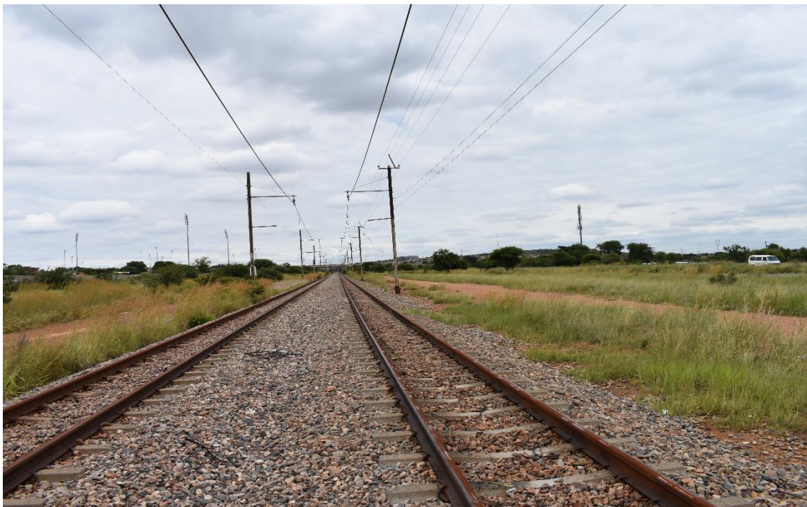
Figure 3: Bridge 1 - Open area
