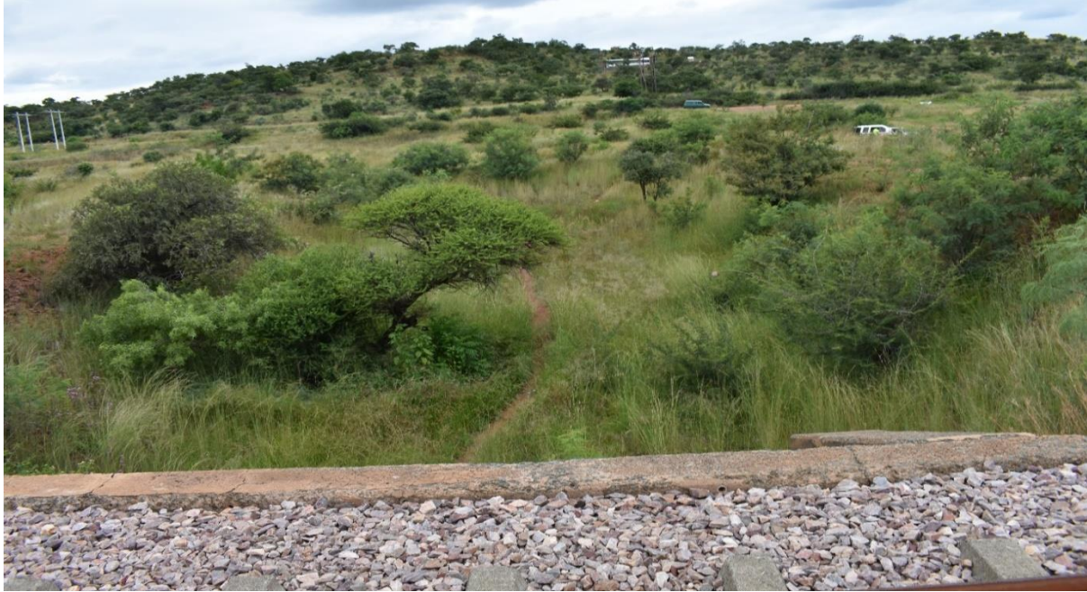
Figure 6: Bridge 2 - Footpath leading away from the stormwater culvert
