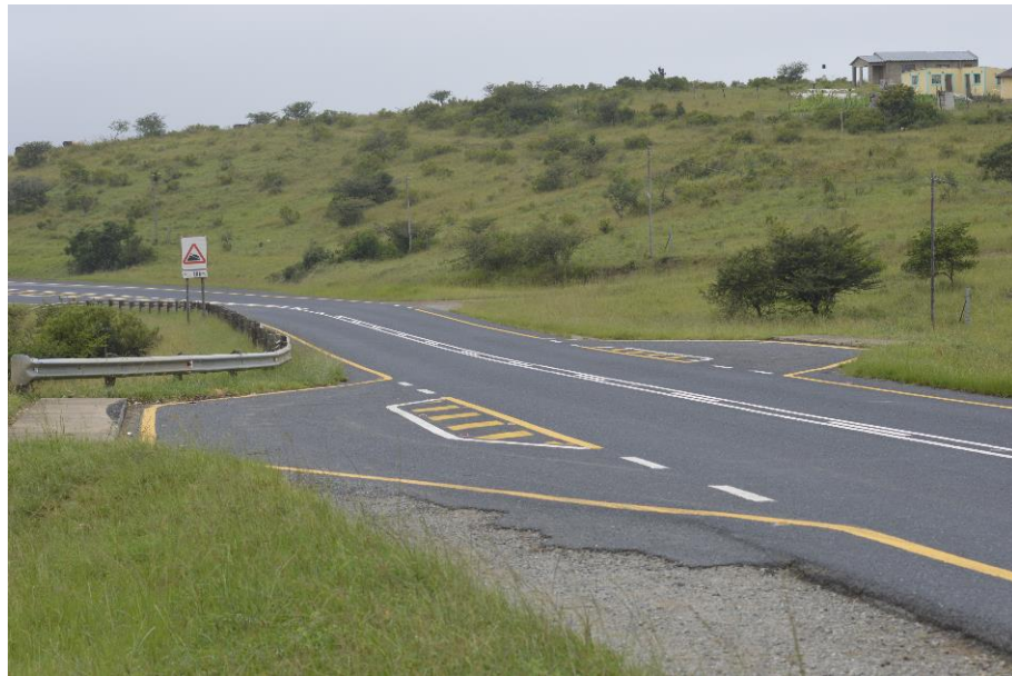
Figure 4.3.2: Existing cross-section bus-bays
