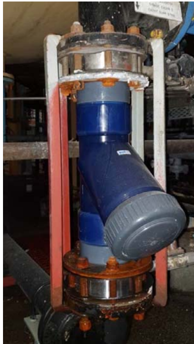
Figure 2: Typical Backwash Outlet U-PVC strainer
