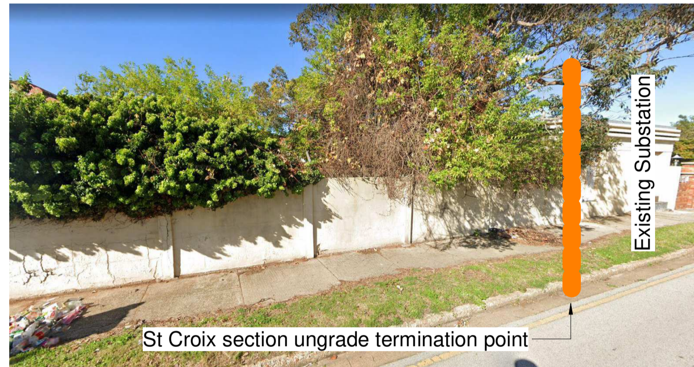
St Croix section ungrade termination point New Security zincalu weld mesh fence to terminate at side of existing substation and continue on the opposite side. New public entrance gate as part of Buckingham Road wall section upgrade.
