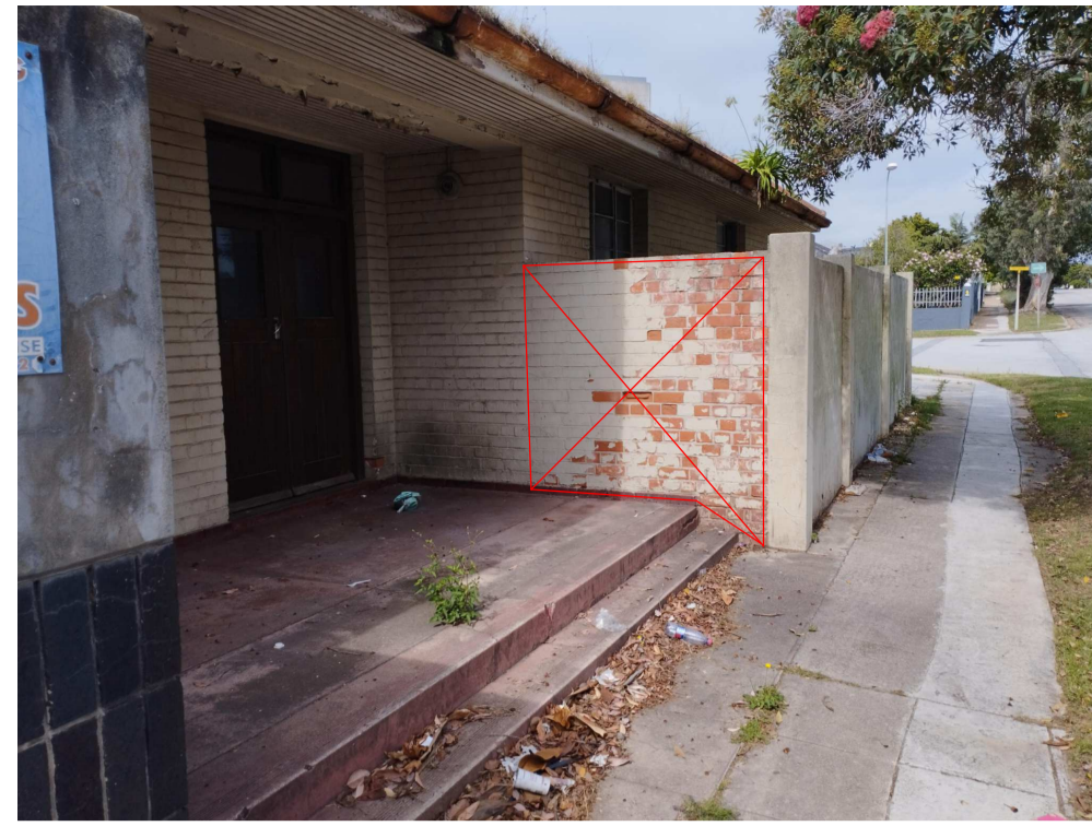
Internal section of wall to be demolished along with boundary wall.
