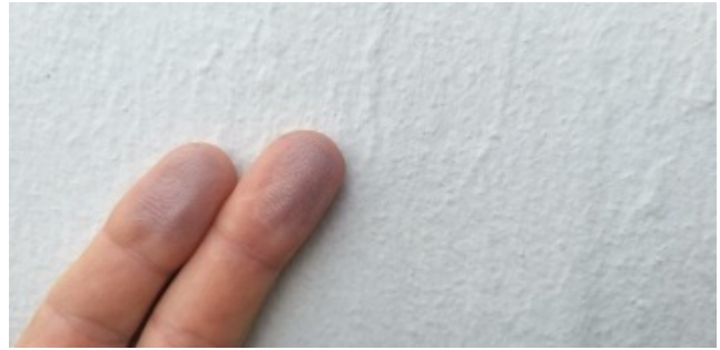
Hydroblast the substrate to remove loose or peeling paint, surface contaminants, or friable materials. If the paint surface is still powdery after Sellotape test, apply a full coat of plaster primer.
