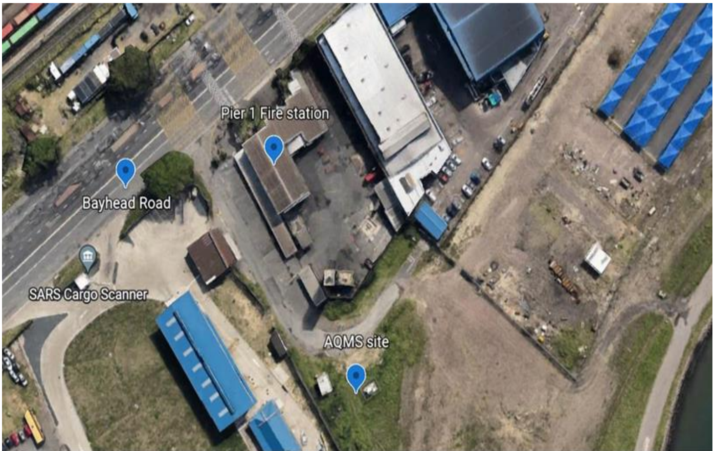
Pier 1 Fire Station (Bayhead Road, Fire station Road)
