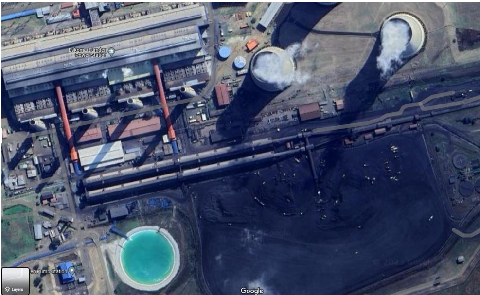
Figure 1: Coal stock yard
