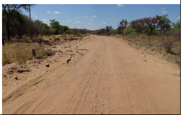
B: Sandy roadway showing water damage
