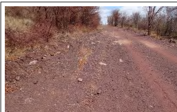
A: Gravel roadway; Big stones on surface
