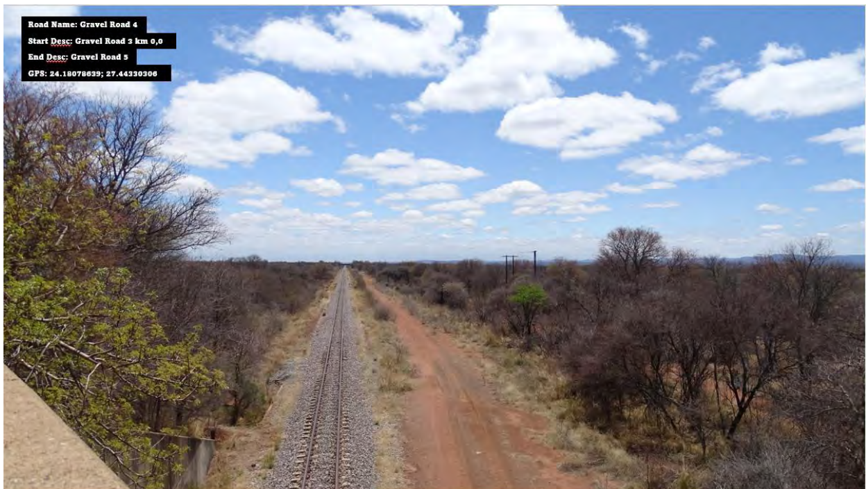
Photo 3.18: Gravel Road 4 (km 12.2): Photo taken facing the North-direction
