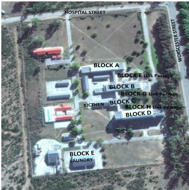
Image 1: Andries Vosloo Hospital, indicating blocks to be renovated
