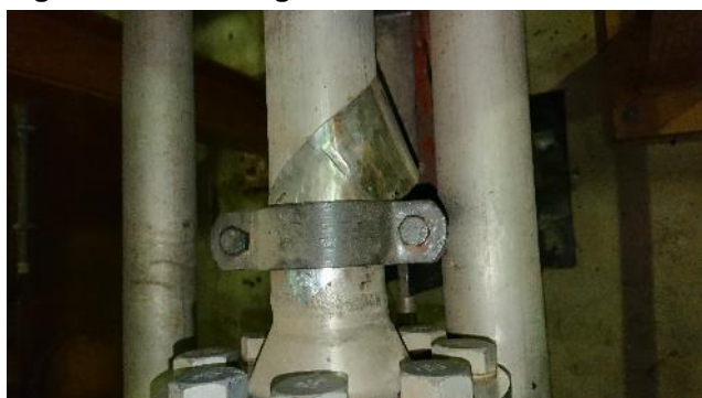
Figure 10: Poorly supported pipe
