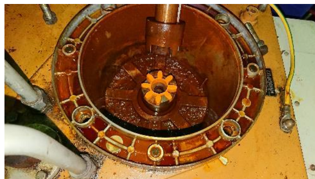
Figure 46: Control oil pump coupling spacer
