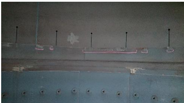
Figure 288: Exhaust – example of crack
