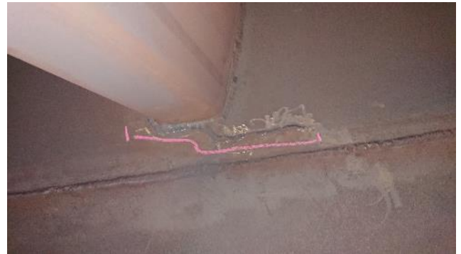
Figure 299: Exhaust – example of crack
