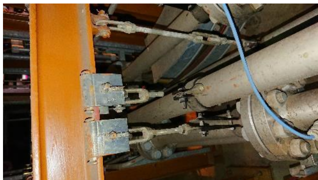
Figure 9: Losse pipe support
