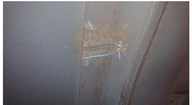
Figure 271: Exhaust – example of crack
