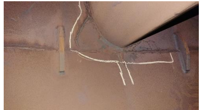
Figure 295: Exhaust – example of crack
