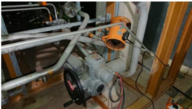
Figure 34: VIGV commander actuator
