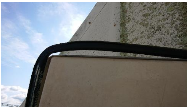
Figure 72: Door seal
