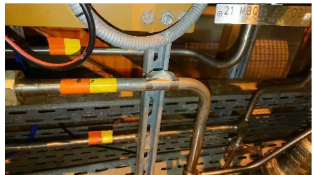
Figure 60: Loose pipe support
