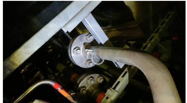
Figure 59: Loose pipe support
