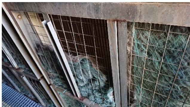
Figure 63: Coalescing filters
