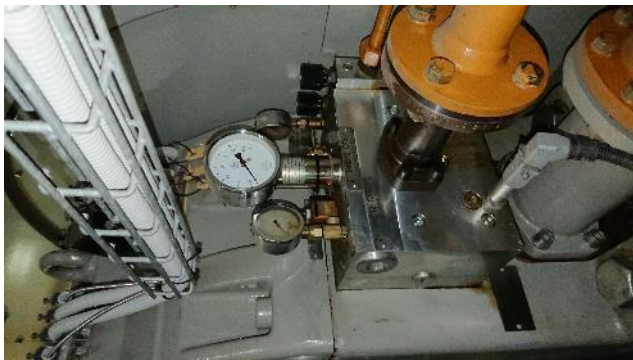
Figure 31: Generator EE bearing
