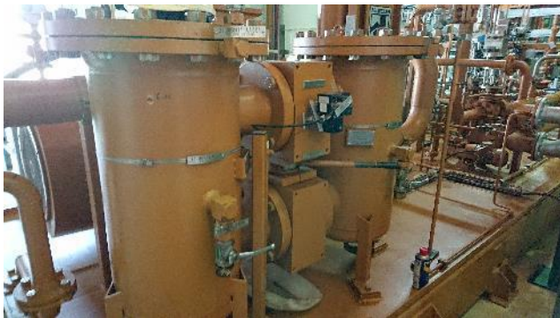
Figure 15: Fuel oil skid
