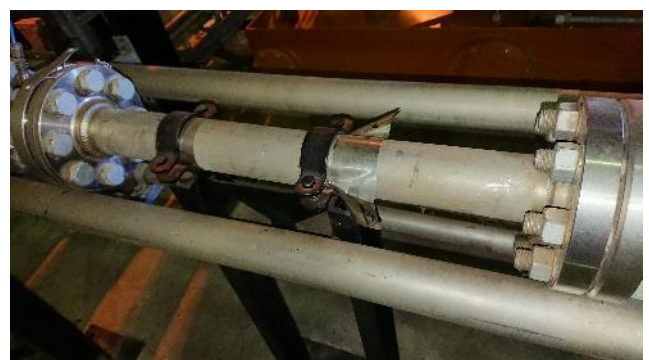
Figure 8: Incorrect pipe support
