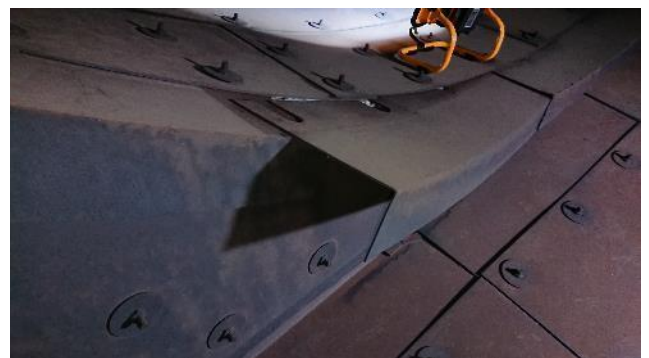
Figure 286: Loose cladding
