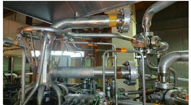
Figure 22: Resonating pipework
