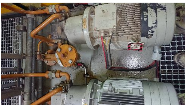
Figure 4: Lubricating oil skid
