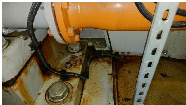
Figure 41: Generator EE bearing
