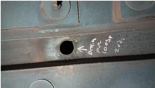
Figure 257: Loose drain pipe
