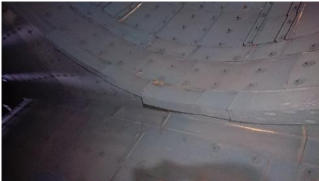
Figure 287: loose cladding
