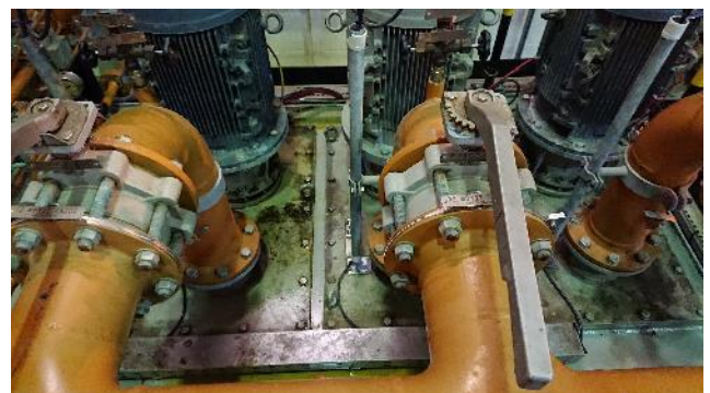
Figure 6: Lubricating oil skid
