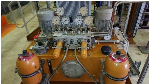
Figure 1: Control oil skid
