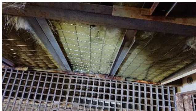
Figure 41: Coalescing filters
