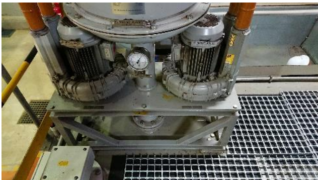
Figure 3: Lubricating oil skid
