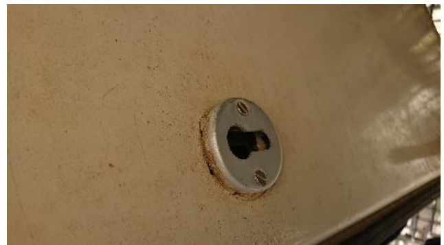
Figure 77: Missing door lock
