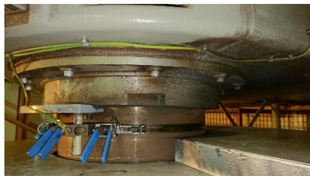
Figure 29: Generator TE bearing
