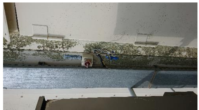
Figure 62: Exposed electrical wires
