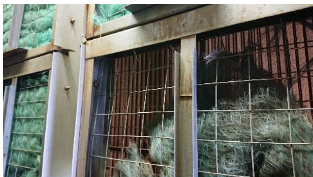
Figure 42: Coalescing filters
