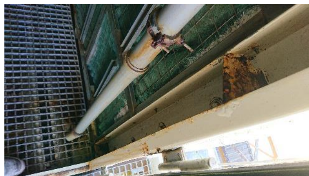
Figure 47: Corroded drain support
