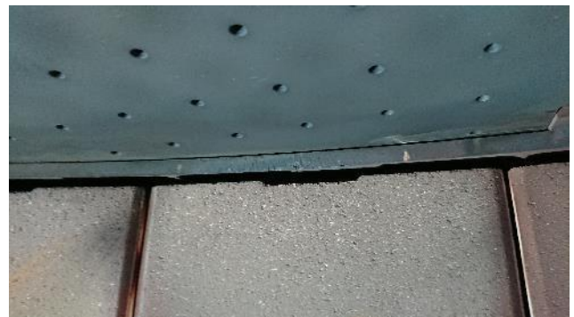
Figure 125: CC1 dome plate support ring
