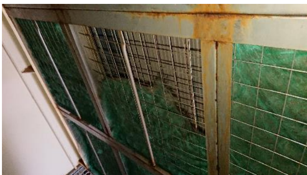
Figure 44: Coalescing filters
