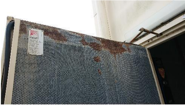
Figure 1: Door rusted
