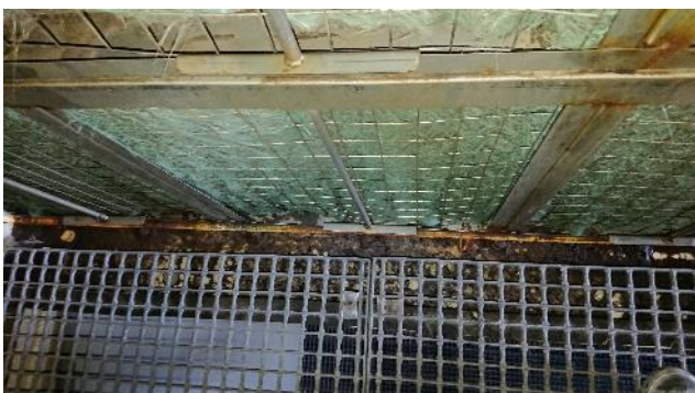
Figure 74: Coalescing filters
