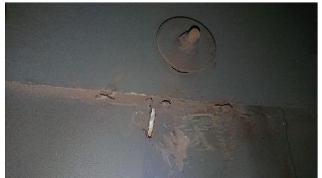
Figure 270: Exhaust – example of crack
