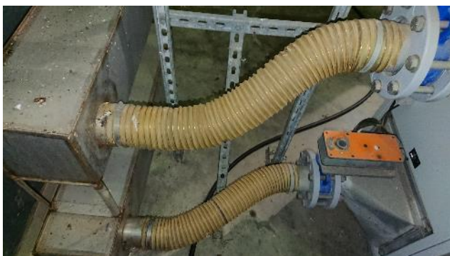
Figure 35: Munters dryer pipes
