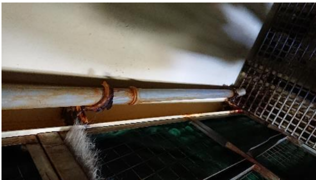
Figure 51: Filter house - corrosion
