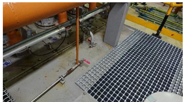
Figure 6: Lubricating oil skid
