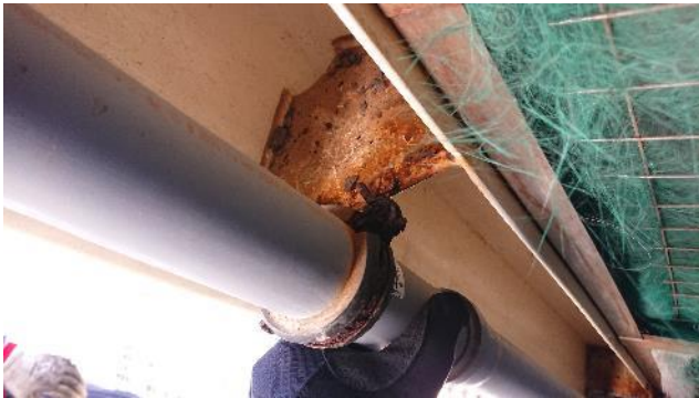
Figure 50: Corroded drain support
