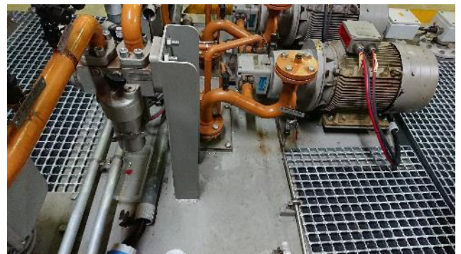
Figure 5: Lubricating oil skid
