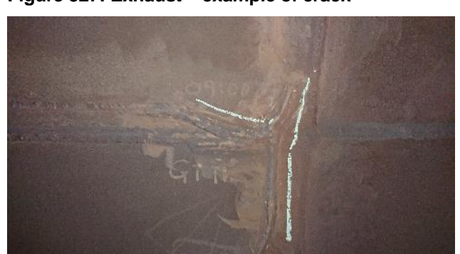
Figure 328: Exhaust – example of crack
