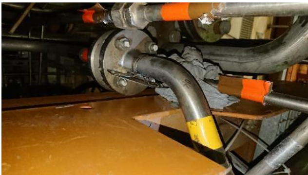
Figure 40: Material used to prevent pipe contact
