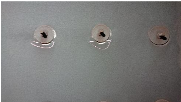
Figure 260: Exhaust – visible insulation
