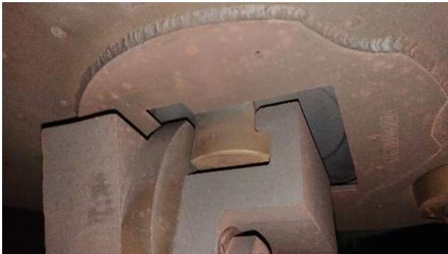
Figure 90: CC2 IC CS support palm
