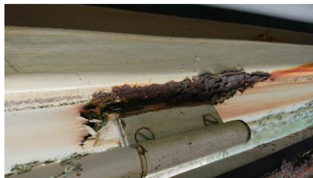
Figure 48: Filter house - corrosion
