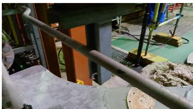
Figure 11: Unsupported pipe
