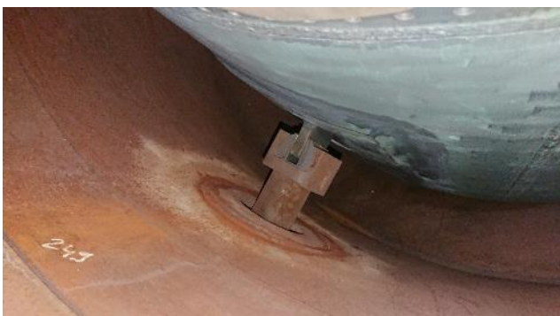
Figure 92: CC2 MC bottom guide
