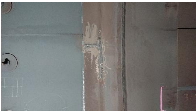
Figure 288: Exhaust – example of crack
