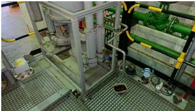
Figure 1: Lubricating oil skid
