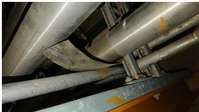
Figure 11: Poorly supported pipe
