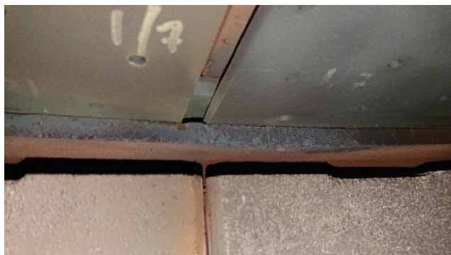
Figure 137: CC1 dome plate support ring
