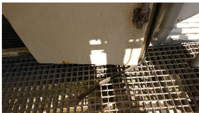
Figure 43: Loose door seal
