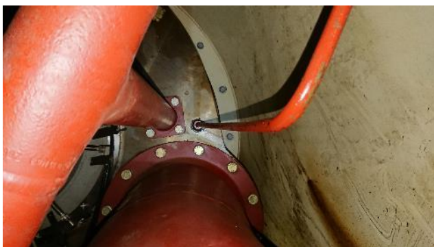
Figure 36: Compressor inlet nose-cone (internal)
